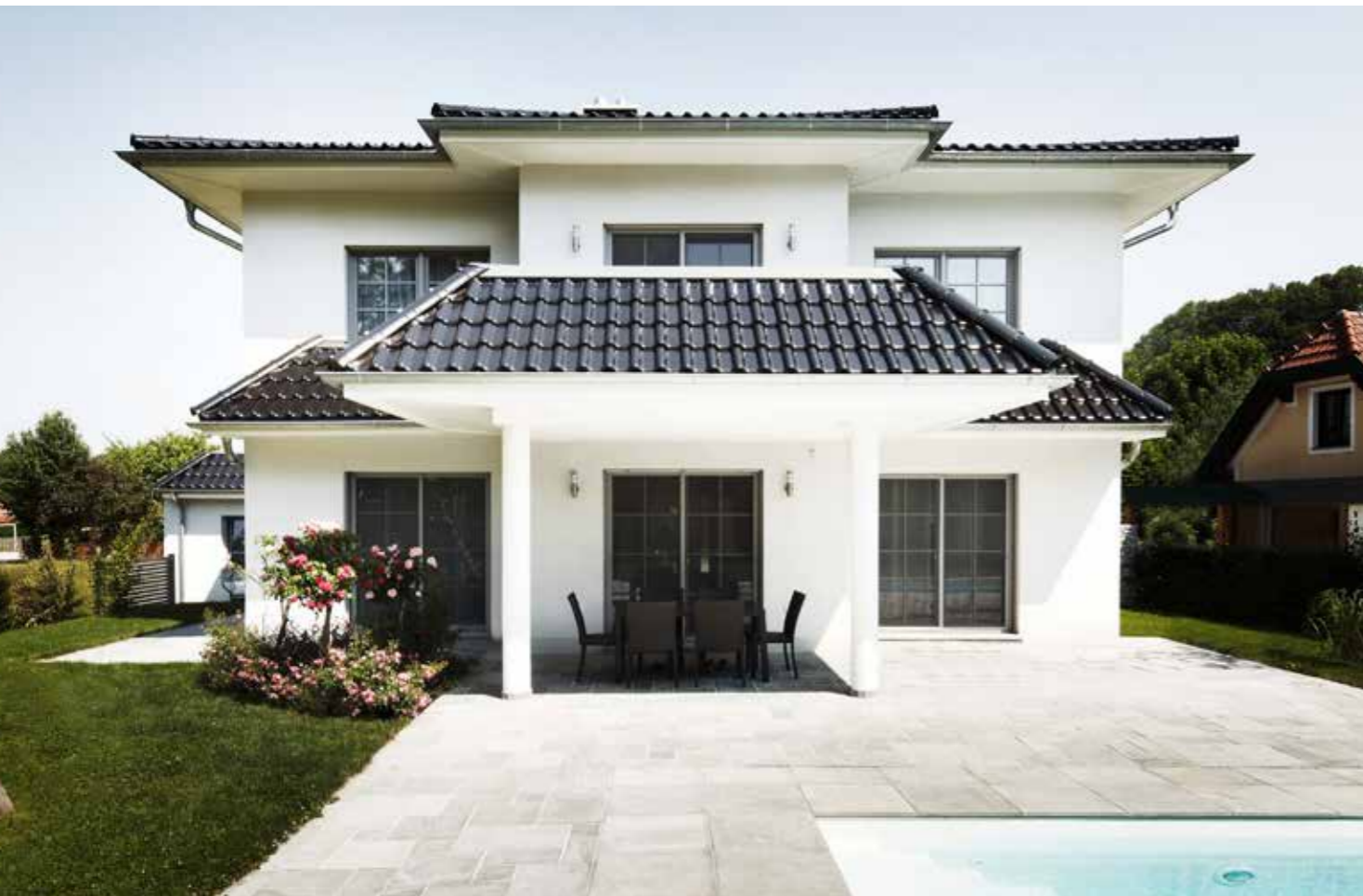
Architect: DI Reinhard Gellner / Eiberbau GmbH, Wels, Austria; photo: Roland Wimmer
