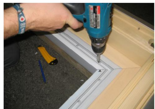
The base-rail and the edge-connector are to be screwed together through the pre-drilled holes using the self-drilling screws 3,5x38mm which are packed with the handle. CAUTION: if the rail is not screwed together in this way, a slot will appear later on due to thermic-expansion of the rail!
