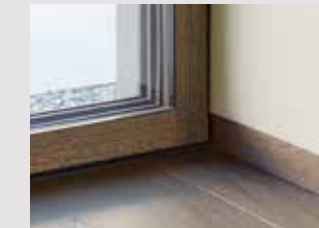
Skirting board with flush wall termination
